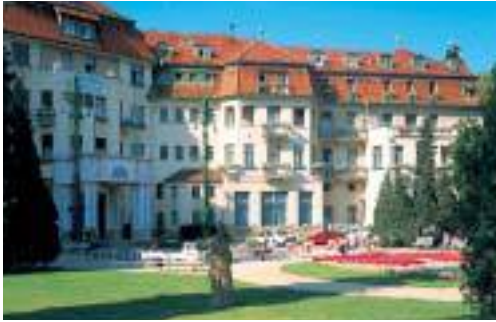
Piešťany - Thermia Palace Spa House
